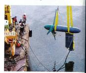
electricity, enough to power 11,000 homes. Six turbines are already installed in New York's East River as part of a tidal power demonstration (Tech Watch, April '07). The new project is the first in which turbines are driven by river currents.
